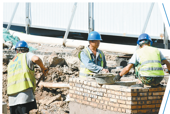
修建雨水窨井
