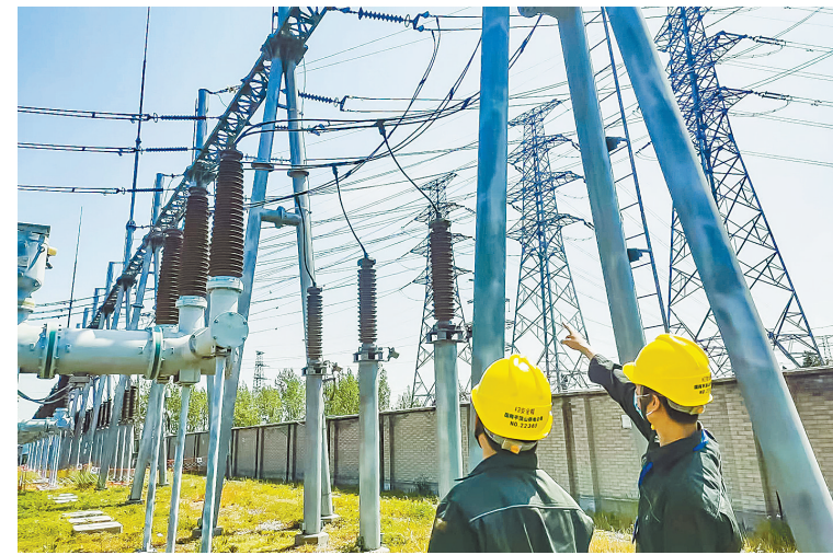
坚守岗位保供电
