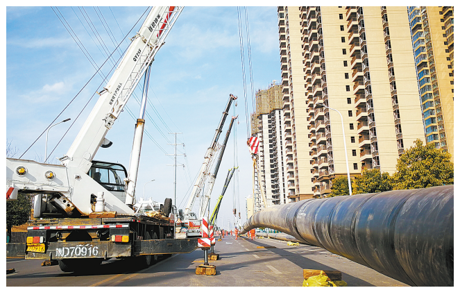
抓紧铺设热力管网
