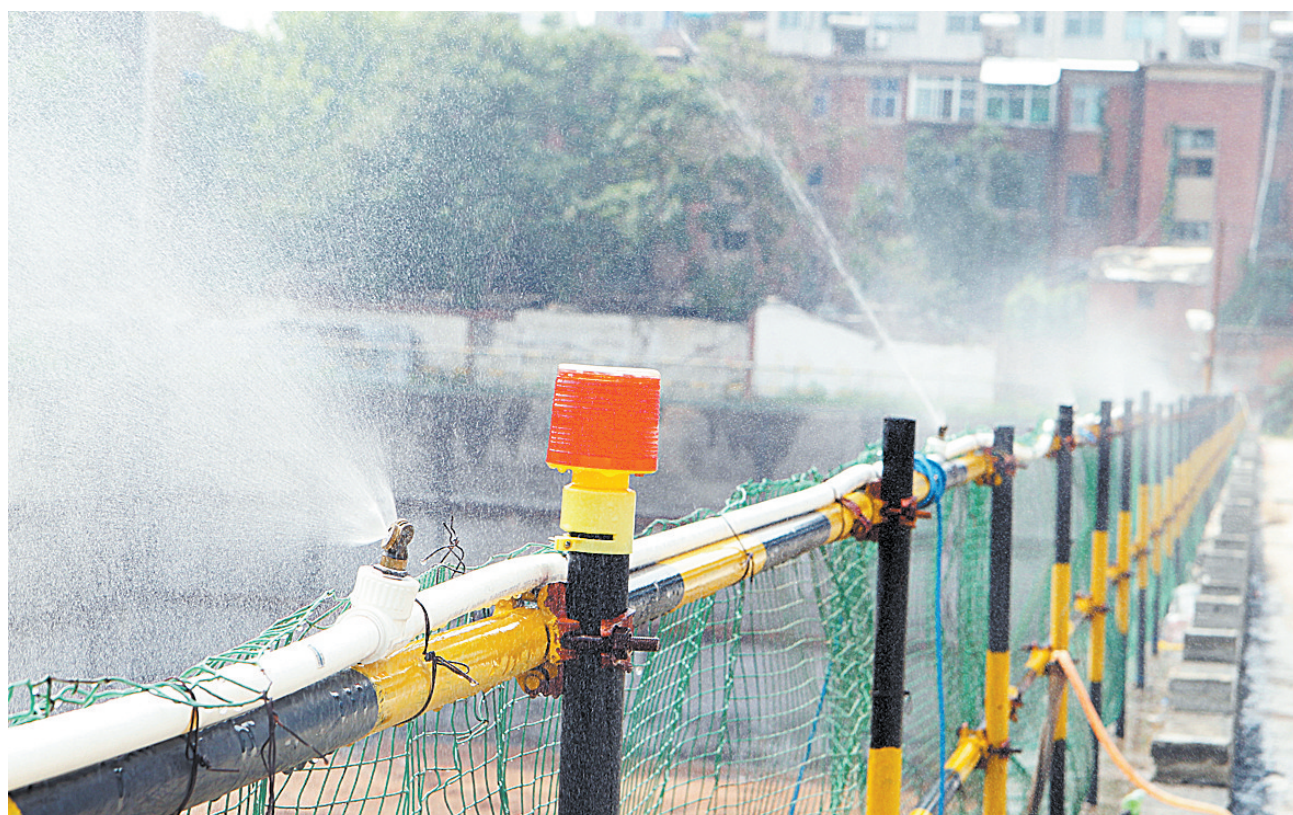
现场喷淋 抑制扬尘
